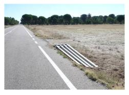
✓ All the components of CROSSAFE are made of materials which can guarantee a service life equal to 25 years in any type of environment, since the elements are made of either reinforced concrete or galvanized steel.
