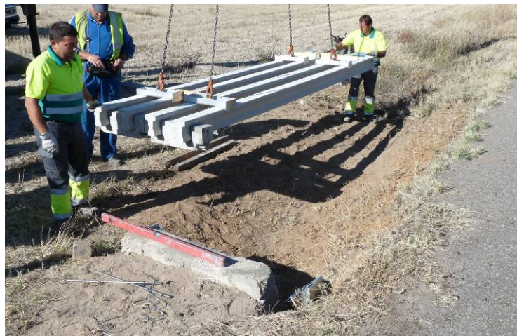
Figure 21.- Manipulation of CROSSAFE device composed of two modules
