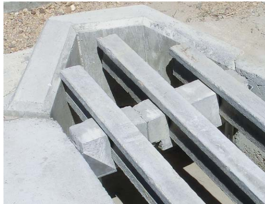
Figure 22.- Installation for culvert-end locations with lateral walls
