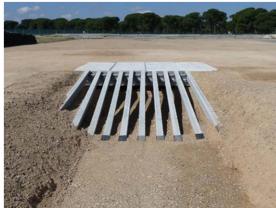
Figure 12.- Ditch configuration of 4 metres width (System made with by five units)
