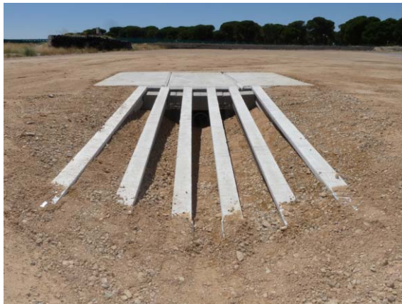
Figure 11.- Ditch configuration of 2,7 metres width (System made by three units)
