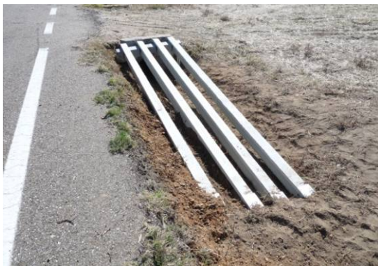
Figure 1.- System installation on standard ditch
