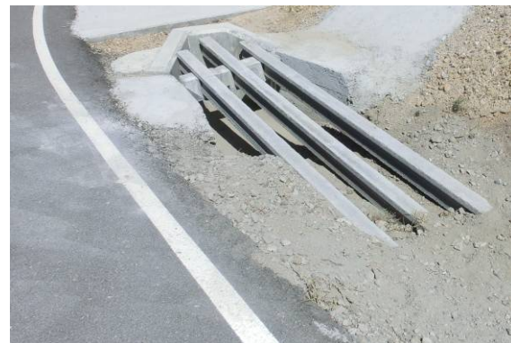
Figure 2.- System installation on a concrete culvert-end
