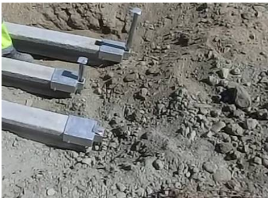
Figure 9.- Anchoring of lower end of longitudinal elements
